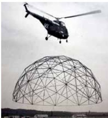
A US Navy helicopter moving a 16,5 m diameter dome 16.5 m, 1954
