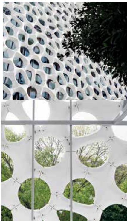
Natural Embellishment, Prosolve 370e a decorative architectural module coated with a superfine titanium dioxide (TiO 2 ), a pollution-fighting technology that is activated by ambient daylight. Installed at Torre de Especialidades, Hospital Manuel Gea Gonzales (Mexico)
