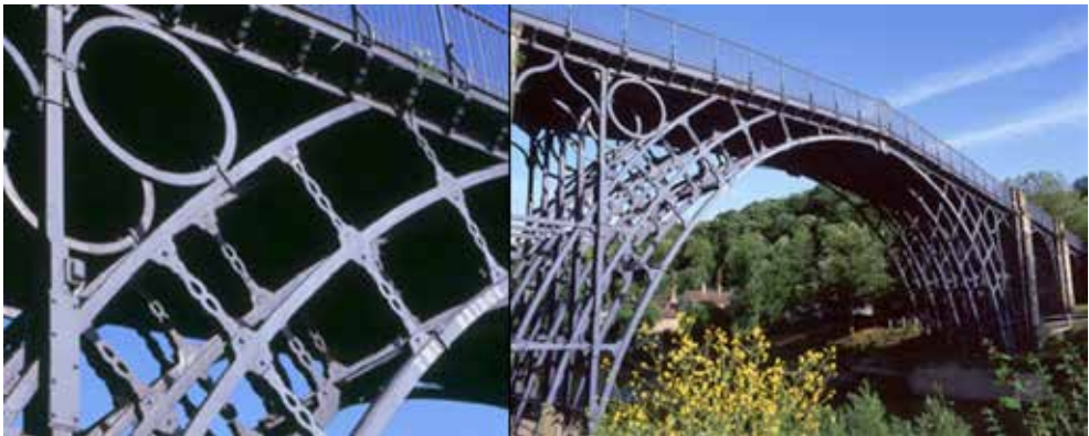
Bridge on River Sever by Abraham Darby III, 1779. A clear example of weaving and how, without scientific knowledge, designer applied the rules of thumbs from other technologies: in this case from the construction of stone arches since cast iron has the same structural behavior of stone.
