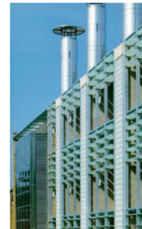
Automated translucent glass louvers at the Environmental Building, Building Research Establishment, Garston, UK (see detailed case study).
