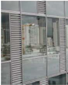
Exterior views of the vertical louvers on the west facade.
