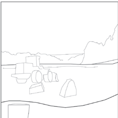
excavator in flattened piazzale area used for temporary storage of marble blocks
