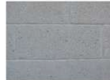
Car ramp wall
