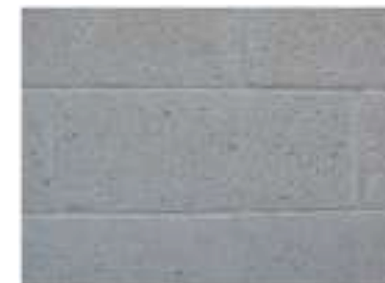
Car ramp wall
